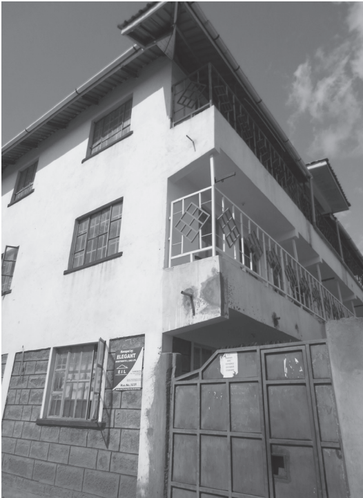
Fig. 14.3. Tanzania-Bondeni. Multi-storey residential building. CLAIRE SIMONNEAU
